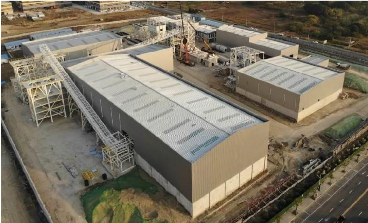
Aerial view of Changzhou construction site, province of Jiangsu, November 2020
