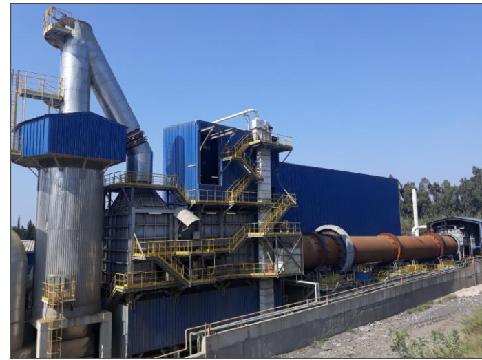
View of the plant and the Waelz kiln
