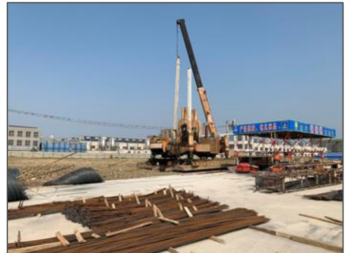
Piling works – Plant buildings
