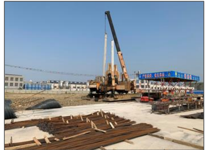
Piling works – Plant buildings
