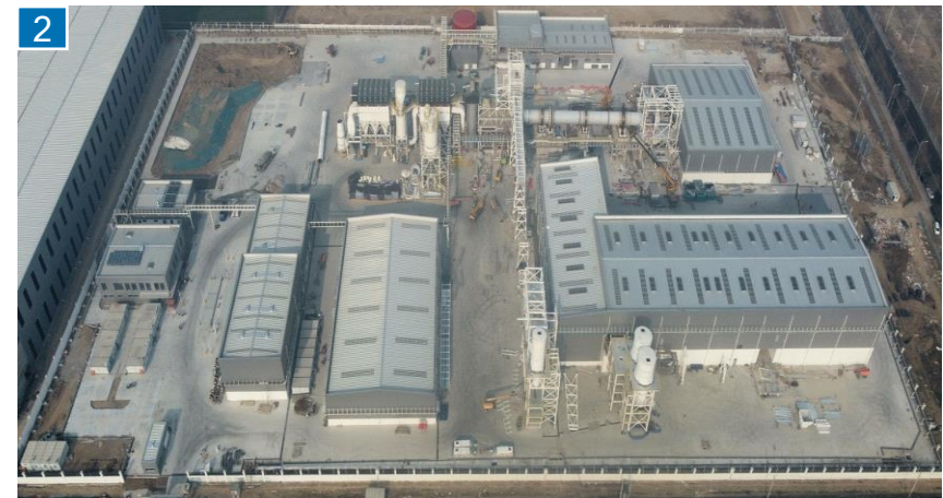
↑ Xuchang plant, construction completed - 27 December 2021
