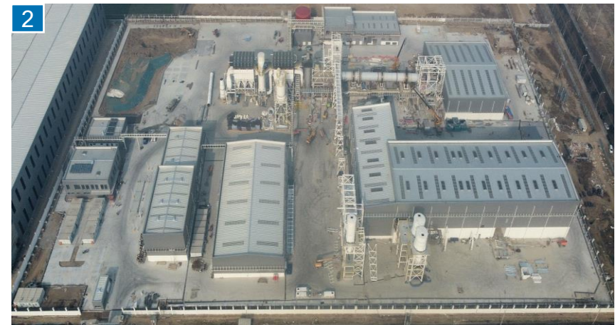
↑ Xuchang plant, construction completed - 27 December 2021
