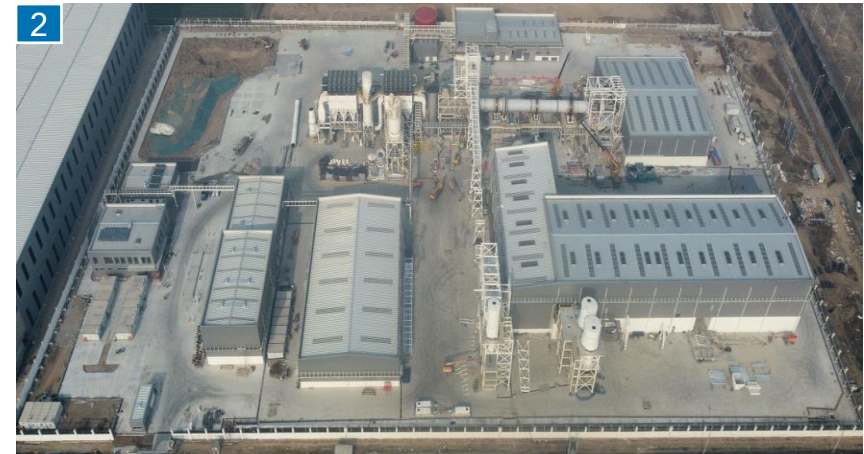
↑ Xuchang plant, construction completed - 27 December 2021
