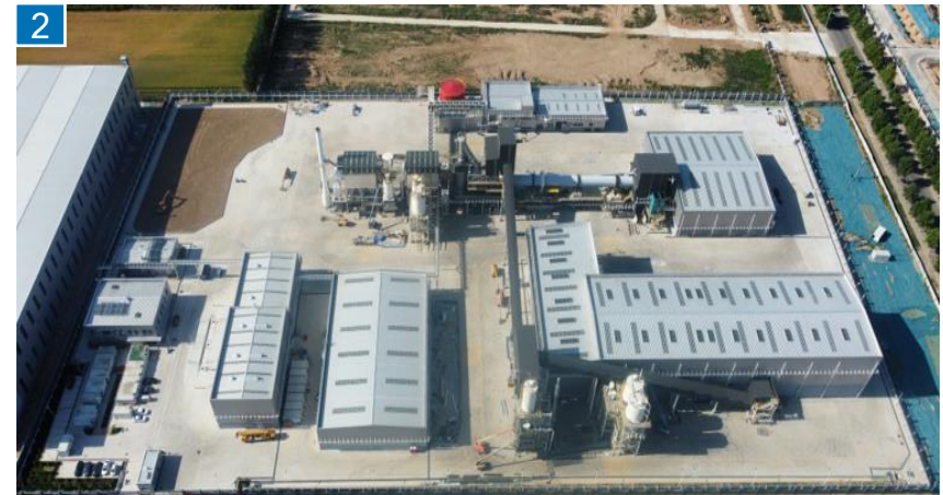
↑ Xuchang plant, mid-May 2022, commissioning
