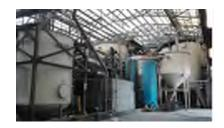
The mixture is pumped into reactors where the aluminous compounds react by maintaining the temperature. The gases produced in the reactors are incinerated in the flare.
